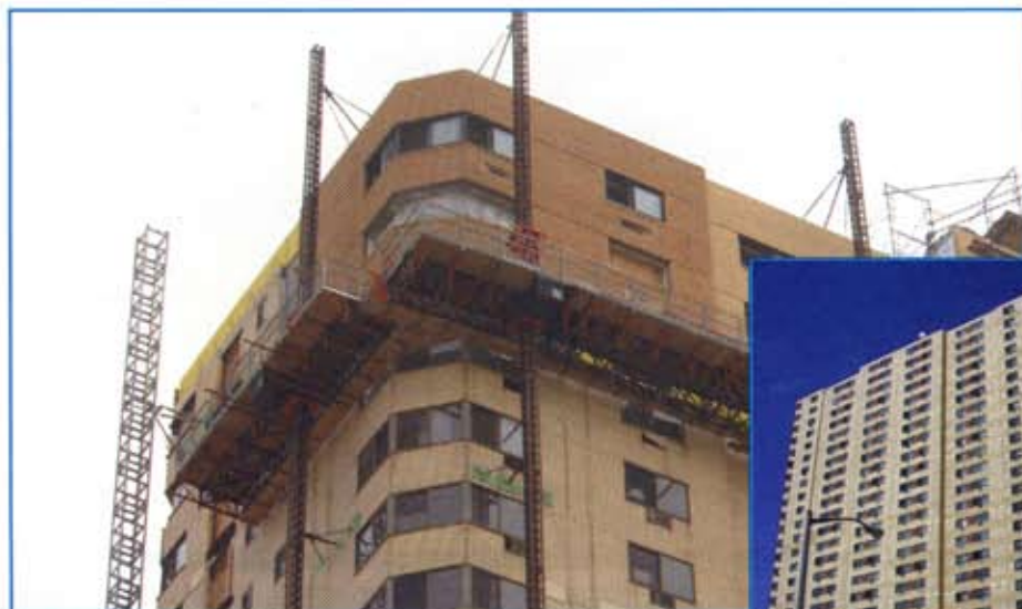
Left - Asbury Tower before restoration. Below right - Asbury Tower after restoration.
