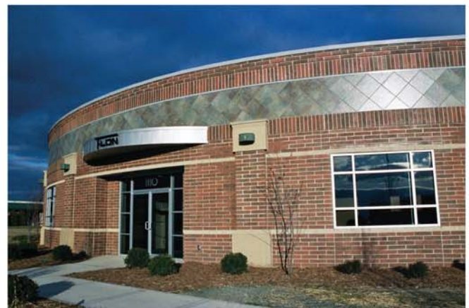
Single Wythe Half-High Construction in Hartland, Wisconsin
