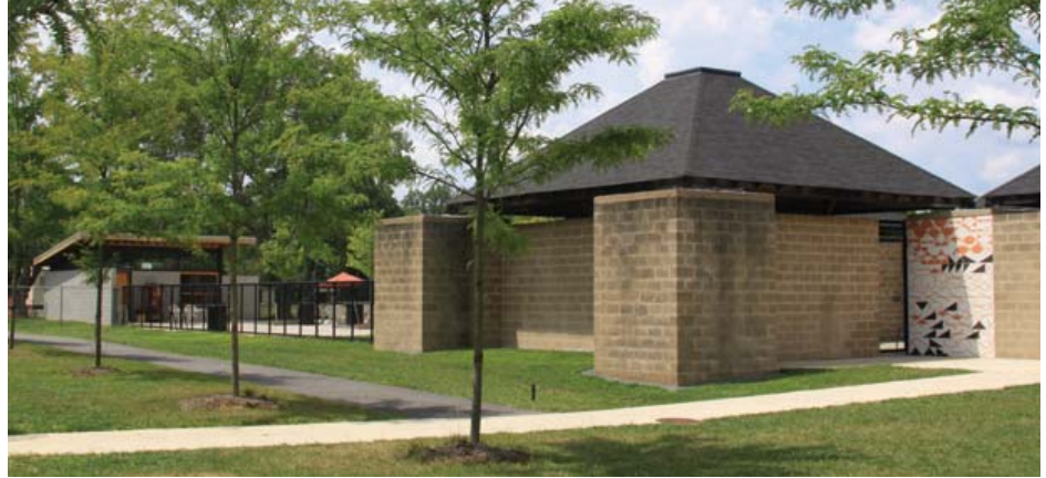
New Jersey's Louis I. Kahn Trenton Bath House uses a unitized flashing system on two new walls.
