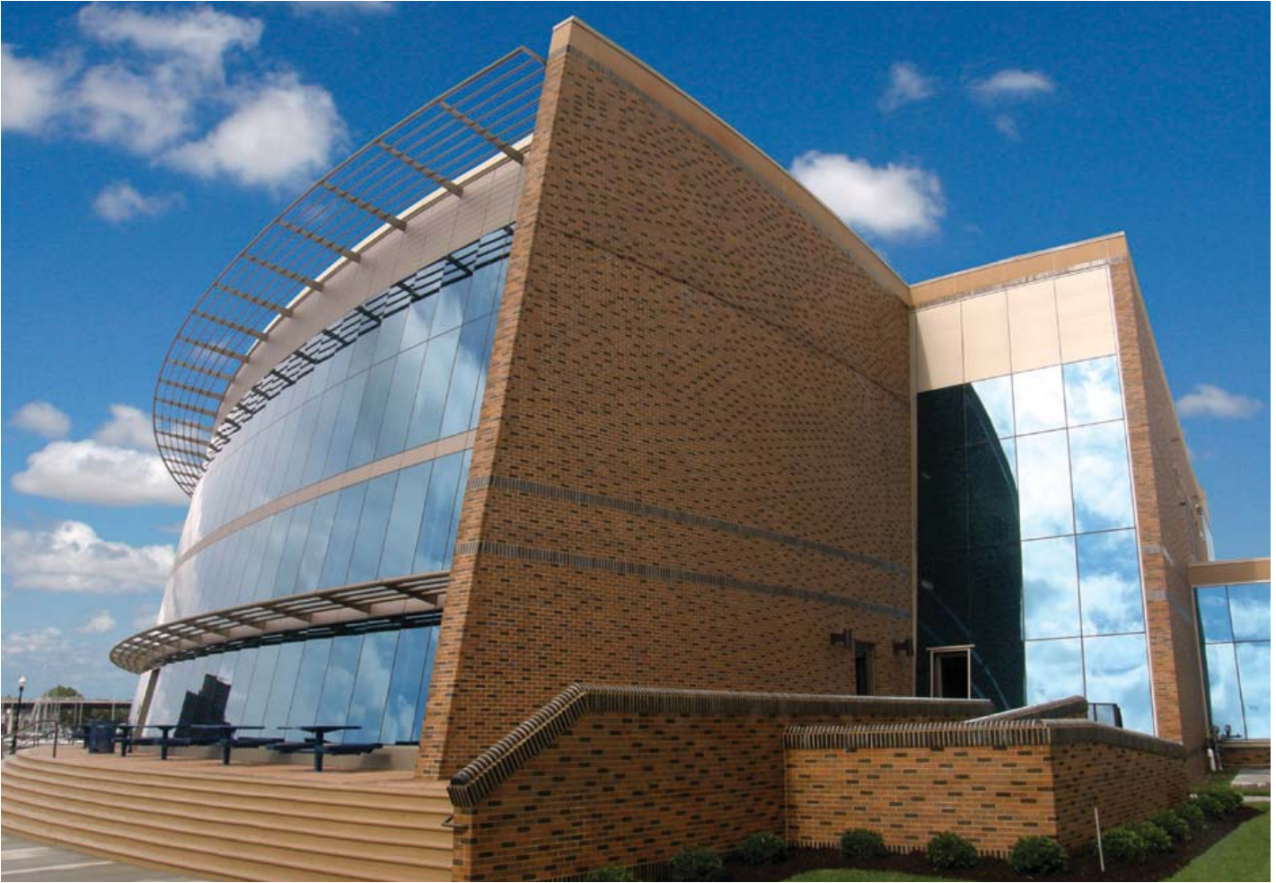
The selection of a unitized flashing system was part of the overall moisture proofing strategy for the Hampton University Student Dining Facility in Hampton, Virginia. Architect of record: Livas Group Architects, P.C. in Norfolk, Virginia.
