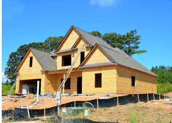
Because house wrap is a non-directional material, when water or water-vapor passes through, it must have the ability to quickly dry to prevent the substrate from becoming saturated. Some critics feel that perforated house wrap products offer a faster drying cycle, while others take the opinion that moisture will not be as likely to get behind the house wrap without holes. The decision to use one product instead of another is based on many geographical and project-specific details.
