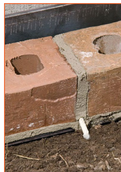
Fig. 7 – Cotton rope wick – not recommended.
