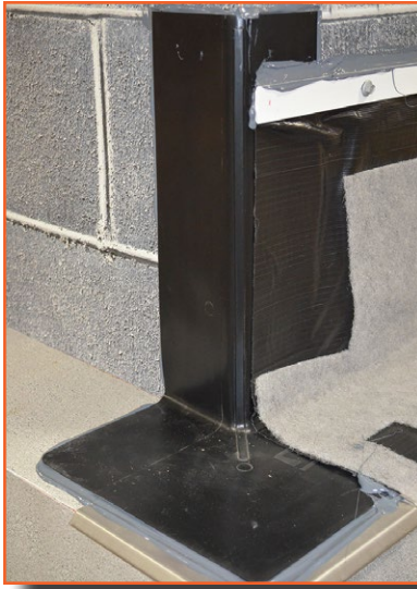
Fig. 4 – Pre-formed one-piece outside corner boot.
