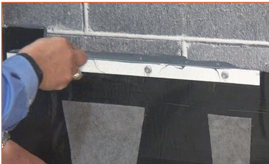
Fig. 6 – Creating a proper seal at the top of a termination bar.
